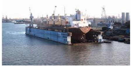
gate on at least one end. The whole thing can be filled with water and sunk in a controlled way. The end gate is then opened so a ship needing repair can be towed into the enclosure. The end gate is then closed and the water pumped out of the dry dock.
